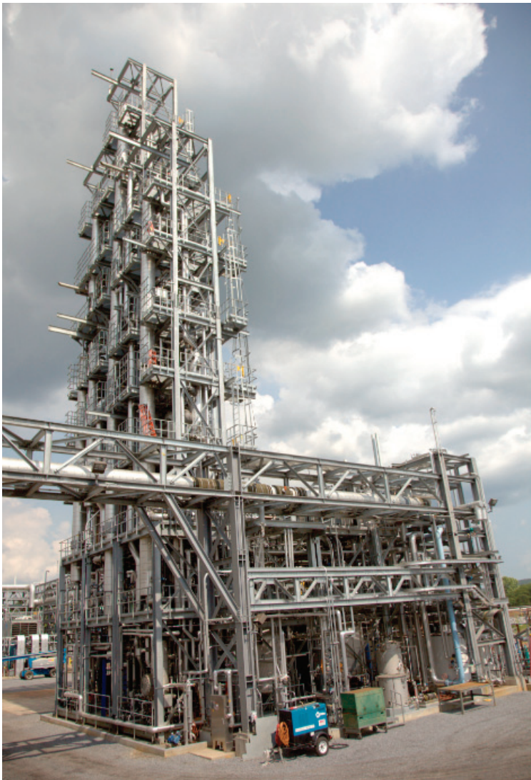
FIGURE 3.6 Conventional amine solvent plant for CO 2 separation at the National Carbon Capture Center in Wilsonville, Alabama. This is a demonstration plant that bridges technologies from the bench scale to the pilot scale, and the absorber unit that is currently in place captures 3,650 tCO 2 /yr. In contrast to the air contactor used for extremely dilute air capture, this flue-gas contactor (absorption column) can be tall for increased CO 2 separation due to the inherent driving force of the flue-gas stream. This image provides an example for dimensional comparison to the DAC plant in Figure 3.5, not a comparison of scale as the annual removal rate by the National Carbon Capture Center is small since it is for demonstration purposes only. SOURCE: Courtesy of Frank Morton, Business Development Manager of the National Carbon Capture Center, Southern Company.
